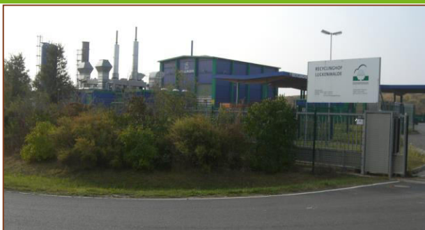
Recyclinghof in Luckenwalde Recycling centre in Luckenwalde
