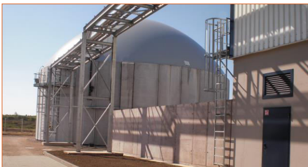
Fermenter Fermentation plant
