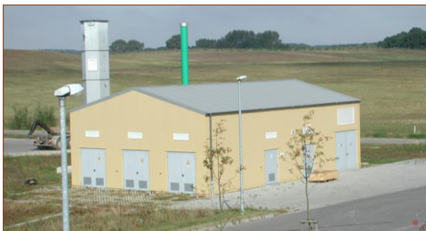
Blockheizkraftwerk (BHKW) Combined heating and power station (CHP)
