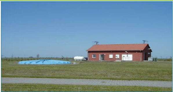
Kläranlage in Breege Purification plant in Breege
